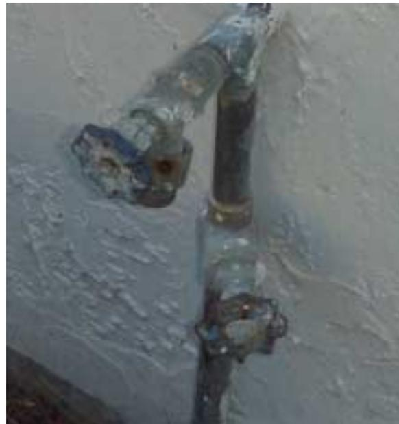
**FIGURE 1: Main Shutoff Valve with Drain Valve at exterior of home.**
