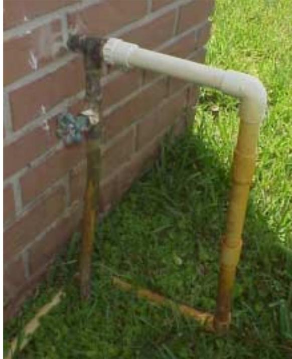
**FIGURE 5: Improper removal of drain valve.**
