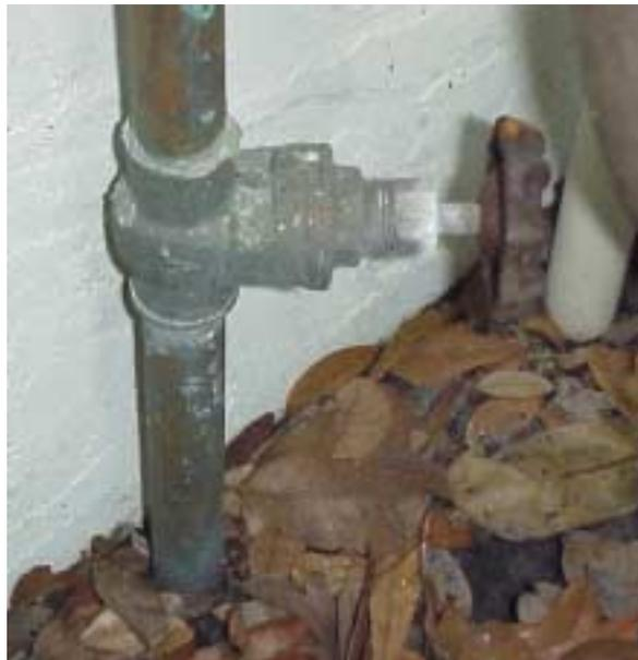
**FIGURE 4: Improperly-Installed Main Shutoff Valve with No Drainage Provisions.**
