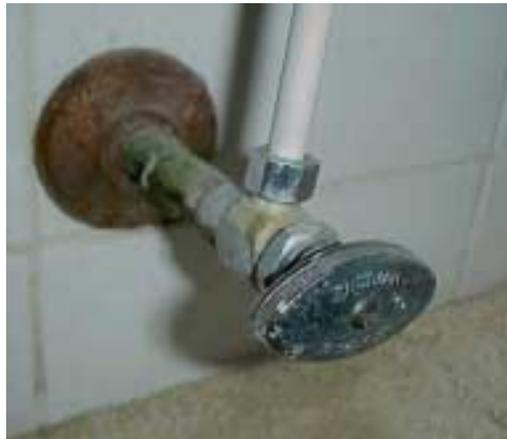
**FIGURE 3: Fixture Shutoff Valve located at the bathroom water closet (toilet).**
